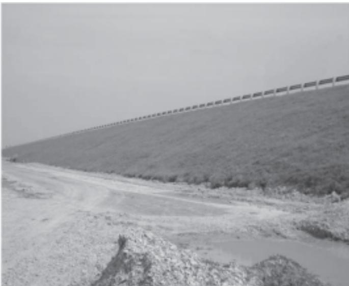
**Fig. 3 : Slope treated with JGT fully covered with vegetation after six months.**
