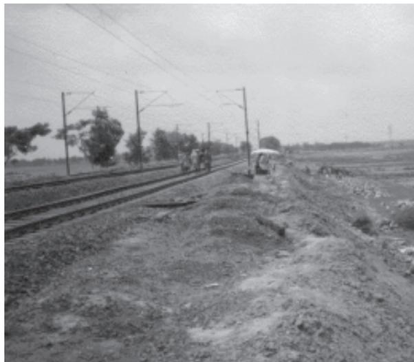
disturbed, side slopes were steeper in places than what the angle of internal friction of this fill could permit, cross-level was not in order, there was creep in formation with erosion of cess along with settlement and surface-soil erosion in slopes. Annex-1 presents the details of the types of problems at different stretches.
