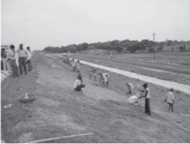
**Fig. 1 : Preparation of slope before laying JGT**
