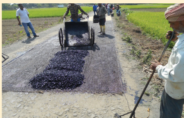
Premix Carpeting on one side of carriage way
