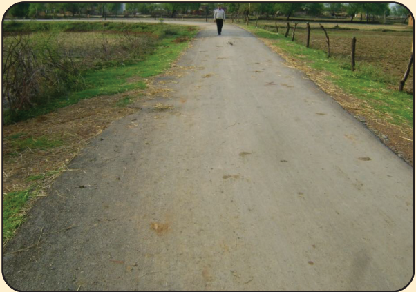
JGT laid section after 26 Months (2009)
