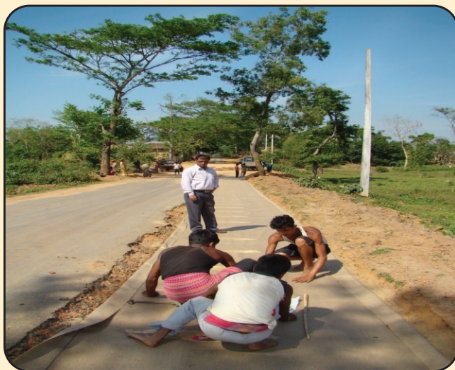
Laying of JGT in widened portion
