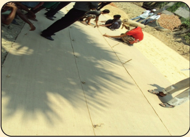
Pegging of overlapped sections of JGT
