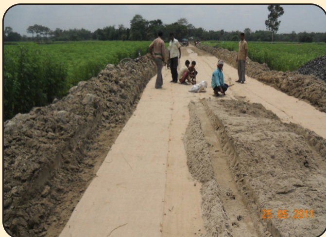
Layer of sand spread over JGT
