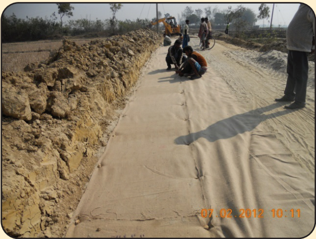
Pegging of overlapped portions of JGT
