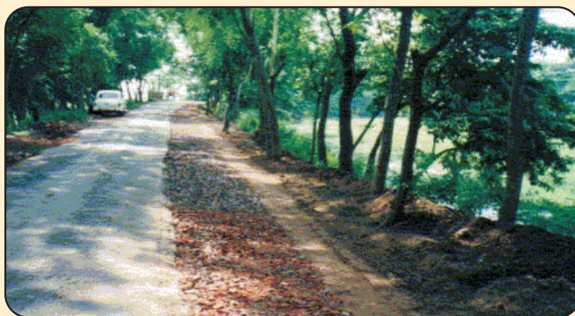
Brick metal laid over JGT
