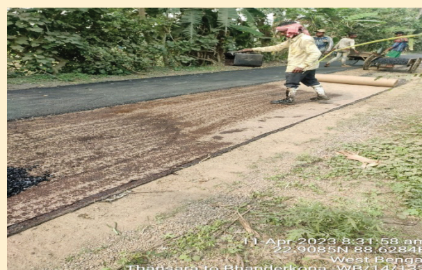
Spreading Prime & Tack Coat on JGT
