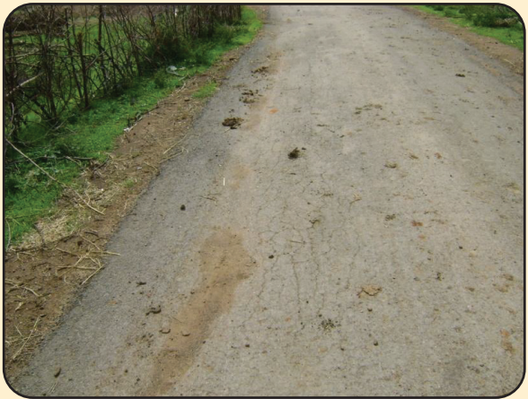
JGT laid section after 26 Months (2009)
