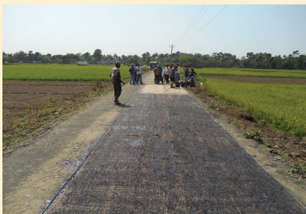
Spreading Prime & Tack Coat on JGT
