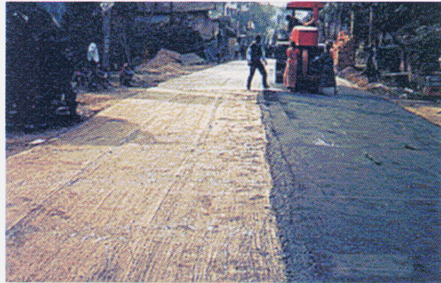
Asphalt Overlay with JAT
