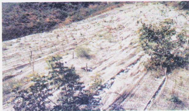
Laying of JGT on the mine spoil
