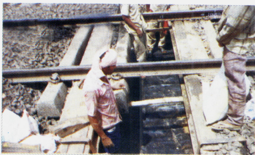
Laying of JGT (Woven & Nonwoven.)
