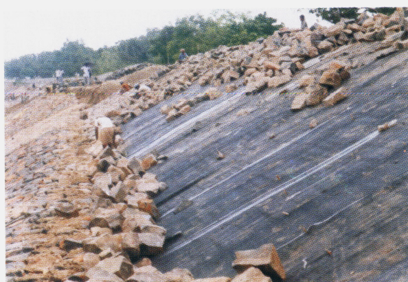
Stone Boulder armour on JGT
