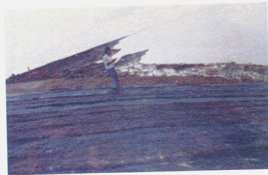
JGT laid on prepared slope of the eroded bank
