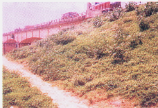
Vegetation on slope after 1 year of laying JGT
