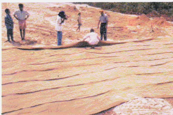
Laying of JGT in Road embankment
