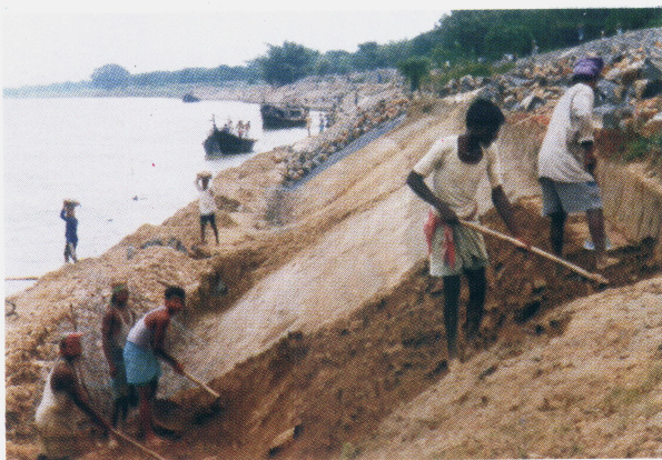
Preparation of embankment slope
