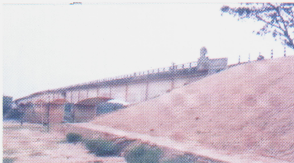
JGT laid on prepared slope of bridge approach road
