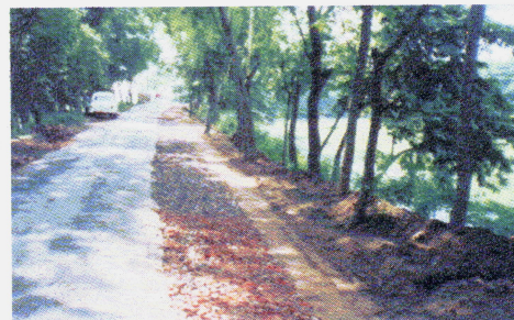
WBM on JGT over brick Soling
