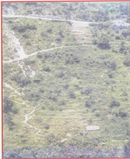
Condition of JGT treated stabilized slope after 9 yrs.
