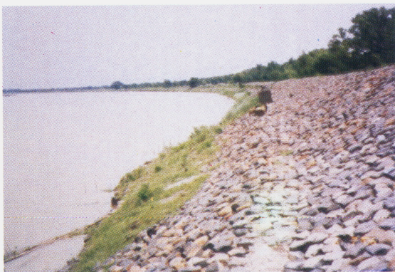
Finished embankment with JGT (after three years of completion).
